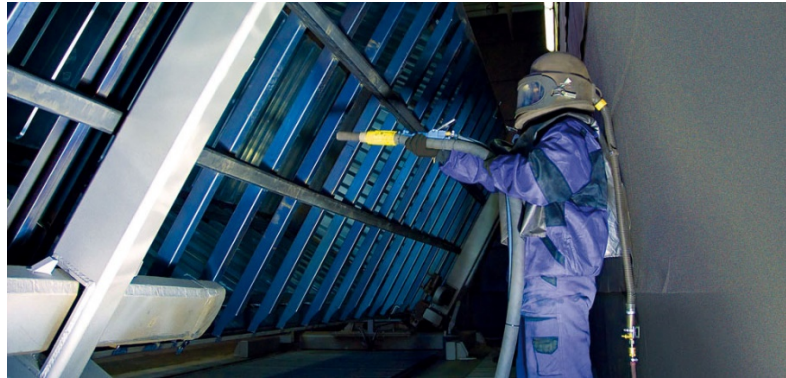
Fig. 3. Manual blasting of the exchange superstructure
